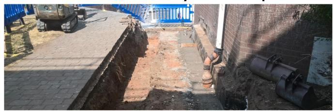
Following a successful tender process Serfis were delighted to be awarded the Access Ramp works at St Johns Campus. The scope of works included excavation, foundations and brickwork. Also installation of slabbed ramp and a low level handrail.
